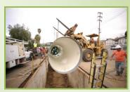
Riverside Public Utilities installed an in-line hydroelectric generator in a 48-inch pipe that utilizes the flow of water to generate electricity. The spherical turbine generates between 2 and 7 kilowatts of energy on a continuous basis, depending on the velocity of water through the pipe, and poses no threat to fish or wildlife.
